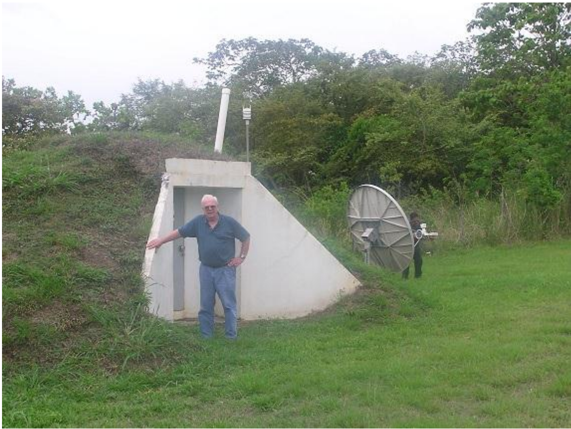
Dave standing in front of University vault while Angel repairs satellite link
